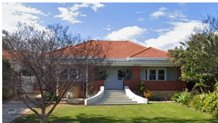
L.J. Walters Architect (at A.M.P. Building) drawing of a 1933 residence at 3 Courthope Street South Perth for Bert and Myrtle Miller. The current stairs at the front are an addition. The entrance was on the left hand side of the house half way along. (Ruth Baird; Google 2024)
